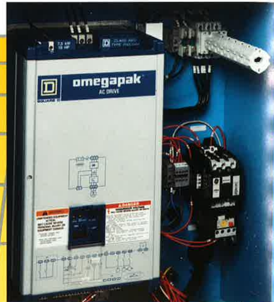
The speed of the motor is controlled by an A.C. inverter to provide infinitely variable band speeds from 40 to 360 fpm (12-110 m/min.) The design assures long life reliability with a minimum of moving parts.
